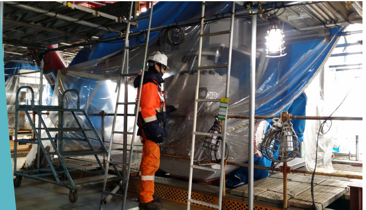
The 17 tonnes ball valve installed on the platform.
